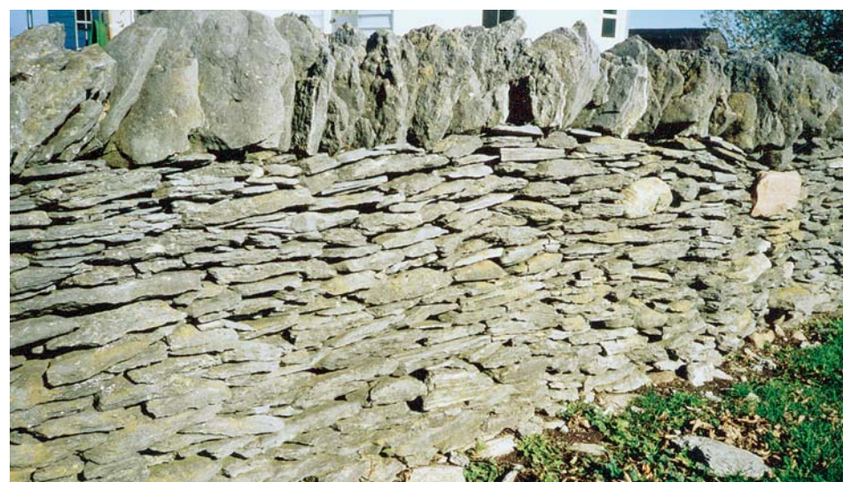
Amherst Island stone fence in good repair
