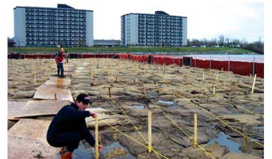
Workers installing mattresses at Belle Park
